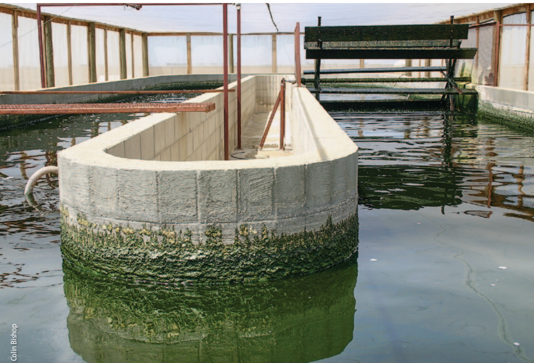
Water treatment facilities at San Joaquin Valley farms. Irrigation water high in nitrogen can contribute to growth of algal blooms, especially blue-green algae.
